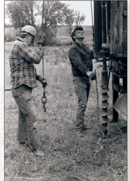
Installation of hydrogeology research site in 1985
