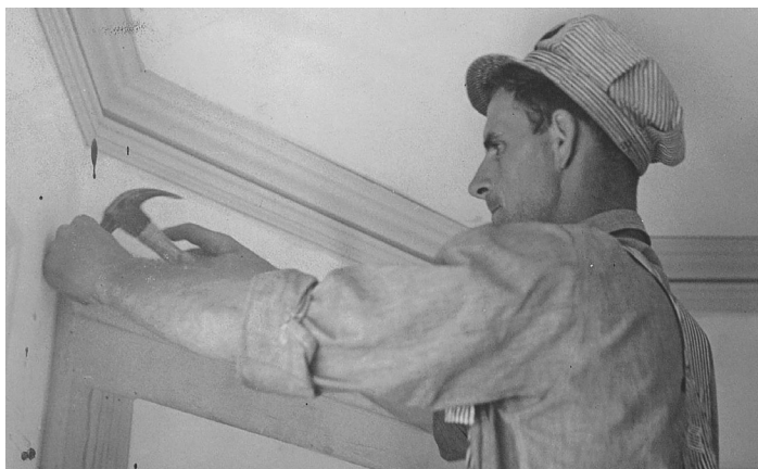
James A. Sublett is working as a carpenter on window trim in 1939, wearing traditional carpenter overalls and a matching soft cap. Today's carpenter in such a situation might sport a hard hat, wear a tool belt over shorts and shirts, and use a nail gun instead of a claw hammer. [Unknown photographer]
