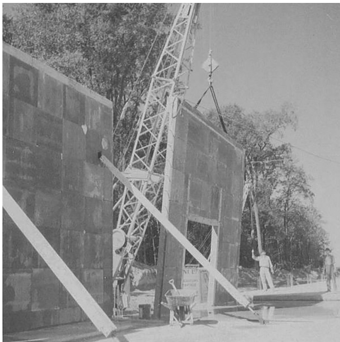
At the Loeb Warehouse in Ottawa a mobile crane lifts a tilt-up wall panel to its final position. The rising panel has an opening in it for access to an outside loading dock. Bracing in the foreground holds a previously lifted panel at the vertical. Note the insulation squares on the inside surface of each panel. [William H. Simon]
